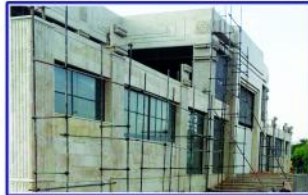
Project title: Mosafer Commercial Complex Site: Southeast side of south terminal Employer: Organization of Investment and Public Participation of the Tehran Municipality Area: 30000 Sq.m Use: Commercial- Parking Position: Excellent Supervision
