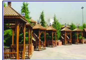
Project title: Setting up Pergola, solar sports equipment, urban furniture, etc. Site: Philosophy Garden, Nowrooz Damavand, and Ab-o-Atash Parks Employer: Abbas Abad Modernization Company Area: 15000 Sq.m Use: Recreational-Welfare Position: Supervision
