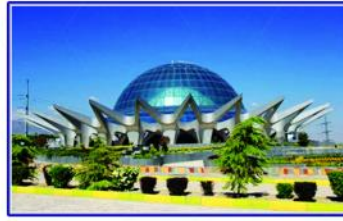
Project title: Enamel Dome (Planetarium) Site: Southern side of Didar Park Employer: Abbas Abad Modernization Company Area: the central sphere with a diameter 30m Use: Cultural-Artistic Position: Supervision
