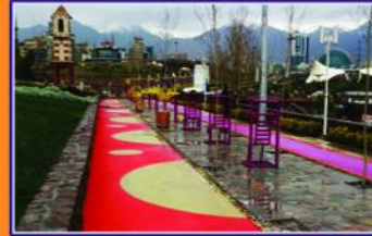
Project title: Constructing bicycle path and children park Site: Philosophy, Nowrooz, and Ab-o-Atash Parks Employer: Abbas Abad Modernization Company Area: 8783 Sq.m Use: Cultural -Recreational Position: Supervision
